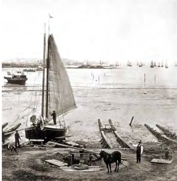
Figure 9. Boatyard at Potrero Point, ca 1870. (Source: Eadweard Muybridge/Bancroft Library and Pier70SF.org)
