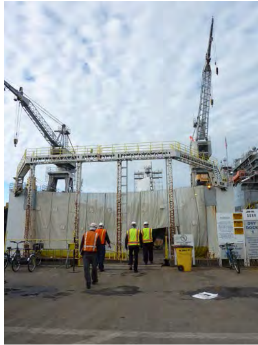
Figure 3. Entrance to Drydock at Pier 70
