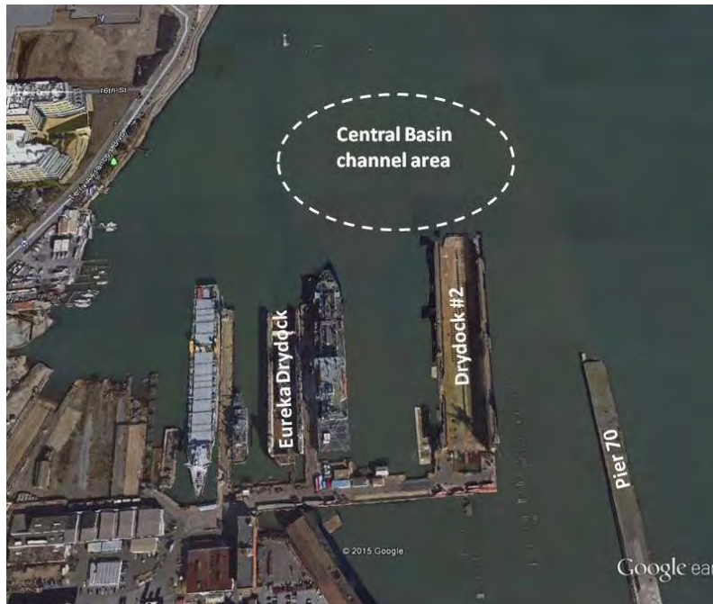
Figure 3. Central Basin channel area and BAE Systems San Francisco Ship Repair dry docks
