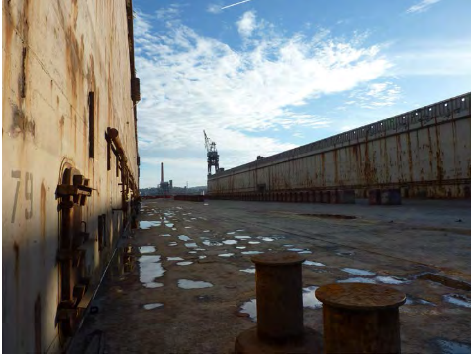
Figure 7. Drydock #2 pictured empty, facing south, with wood and steel pilings used to support ships.
