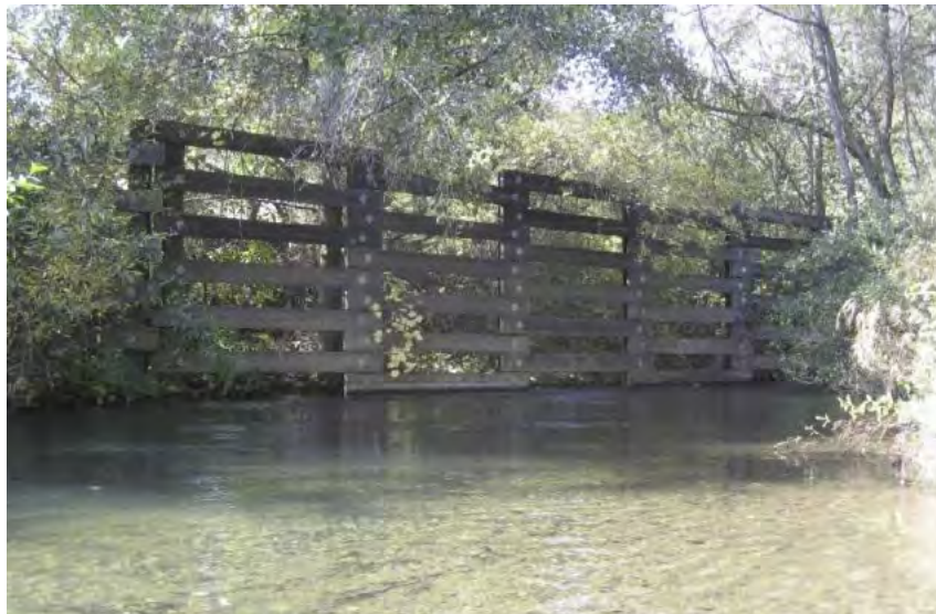
Figure 32. 700 foot board fence in subreach 14a
