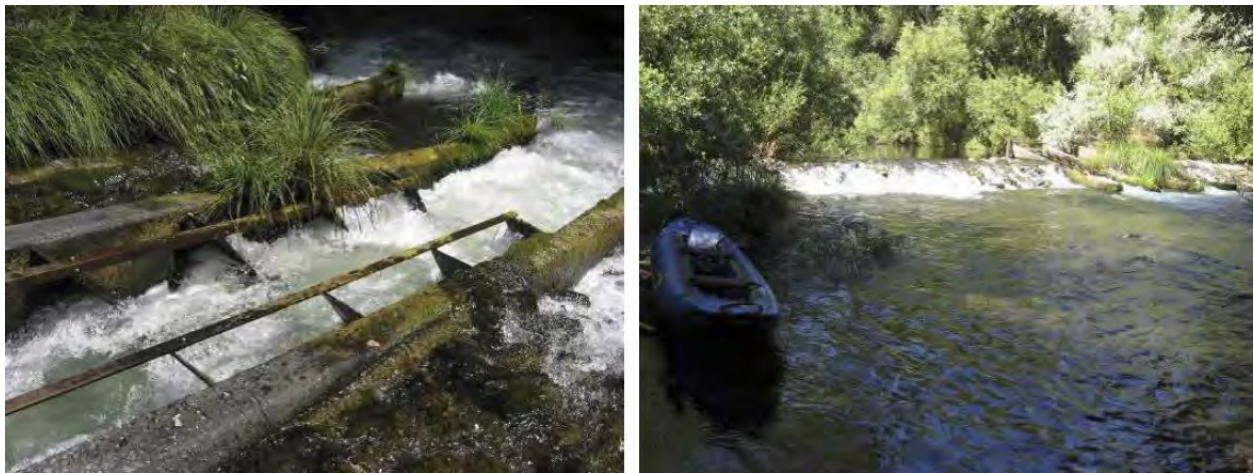
Figure 33. (left) ladder on middle sill, (right) middle sill.
