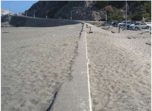
When this photograph was taken in June 2012, sand covered the stairs, bleacher seating, and part of the pedestrian walkway and parking lot along the seawall. The seawall was almost completely buried.
