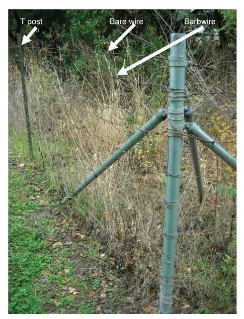
Note: Metal t post with hog wire topped with one strand of barbwire and one strand of bare wire. (typical along most park boundaries)
