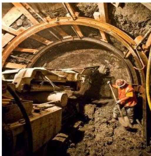
**Figure 2.7-3 Roadheader Excavation with Steel Sets at the Face of a Tunnel**
