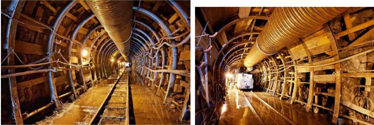
**Figure 2.7-7 Tunnel with Steel Rib and Wood Lagging Initial Support**
