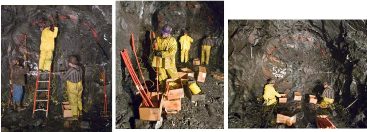
**Figure 2.7-6 a, b, and c—Photographs of Controlled Detonation Preparation**
