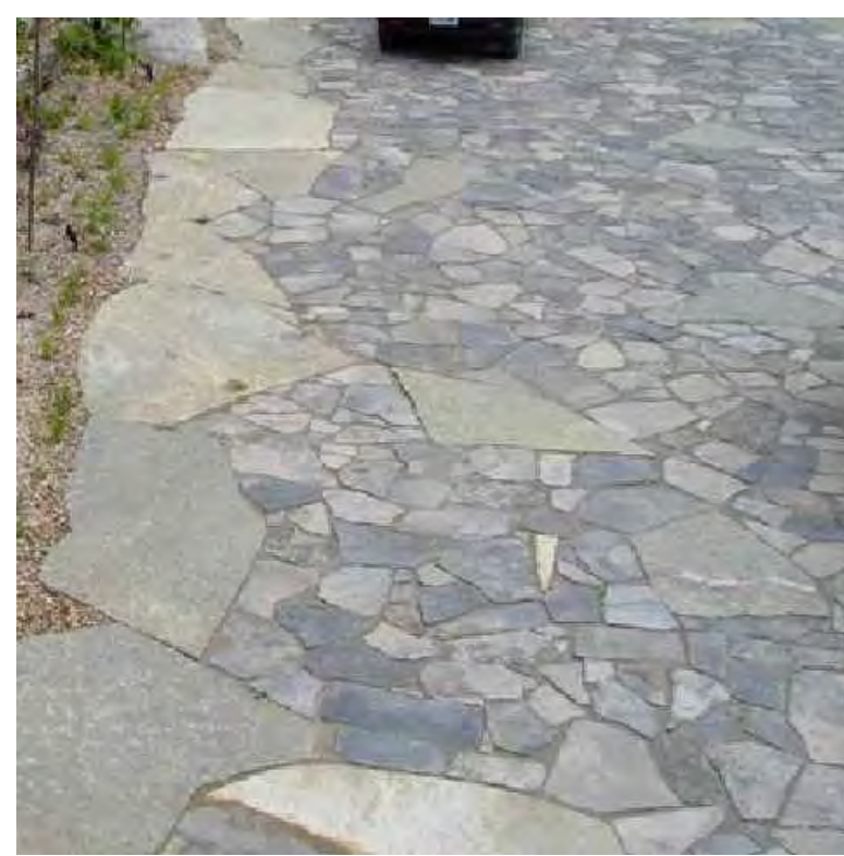
Enhanced Motor Court Paving
