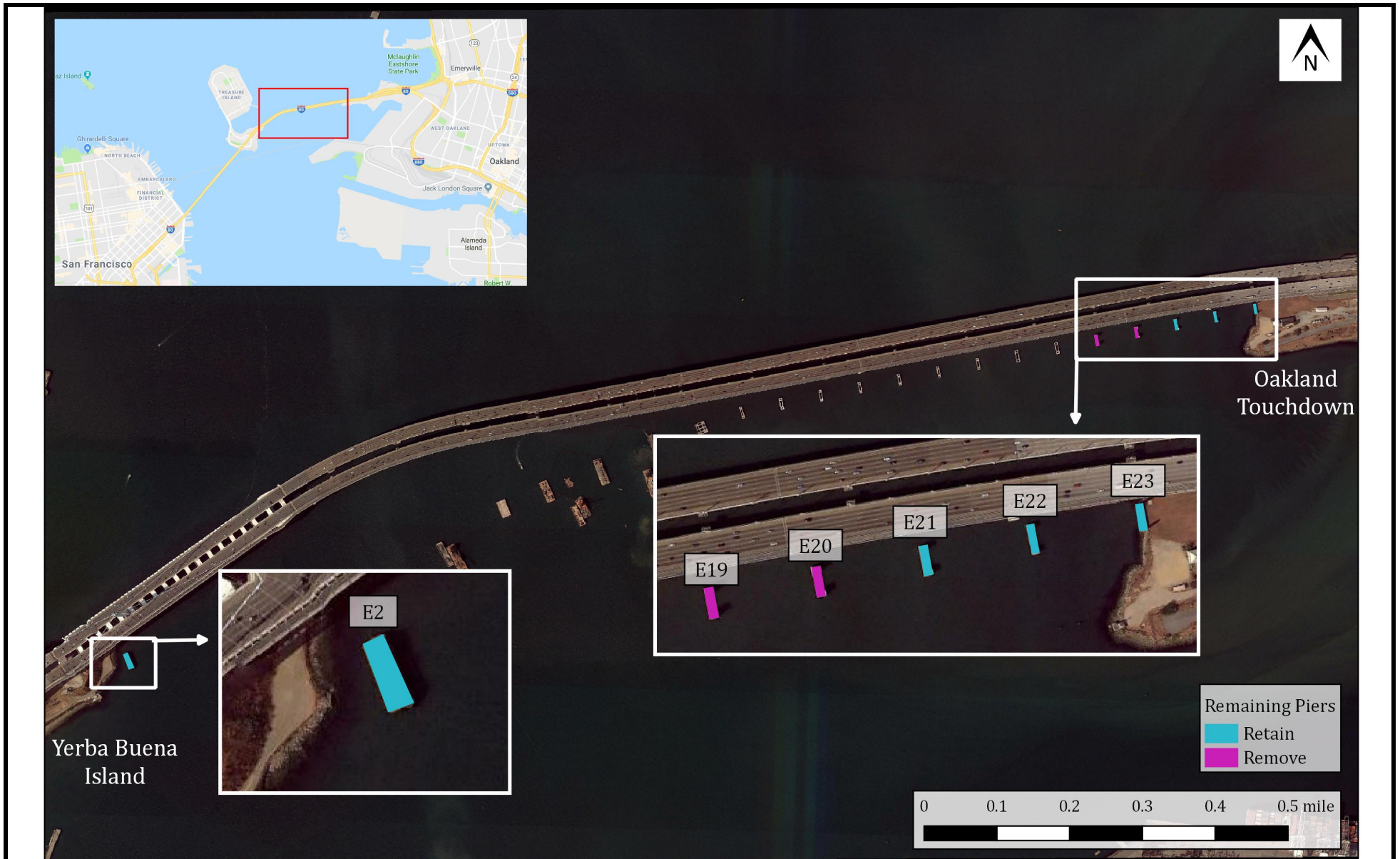
Figure 2. Remaining SFOBB Piers Proposed for Retention and Removal
