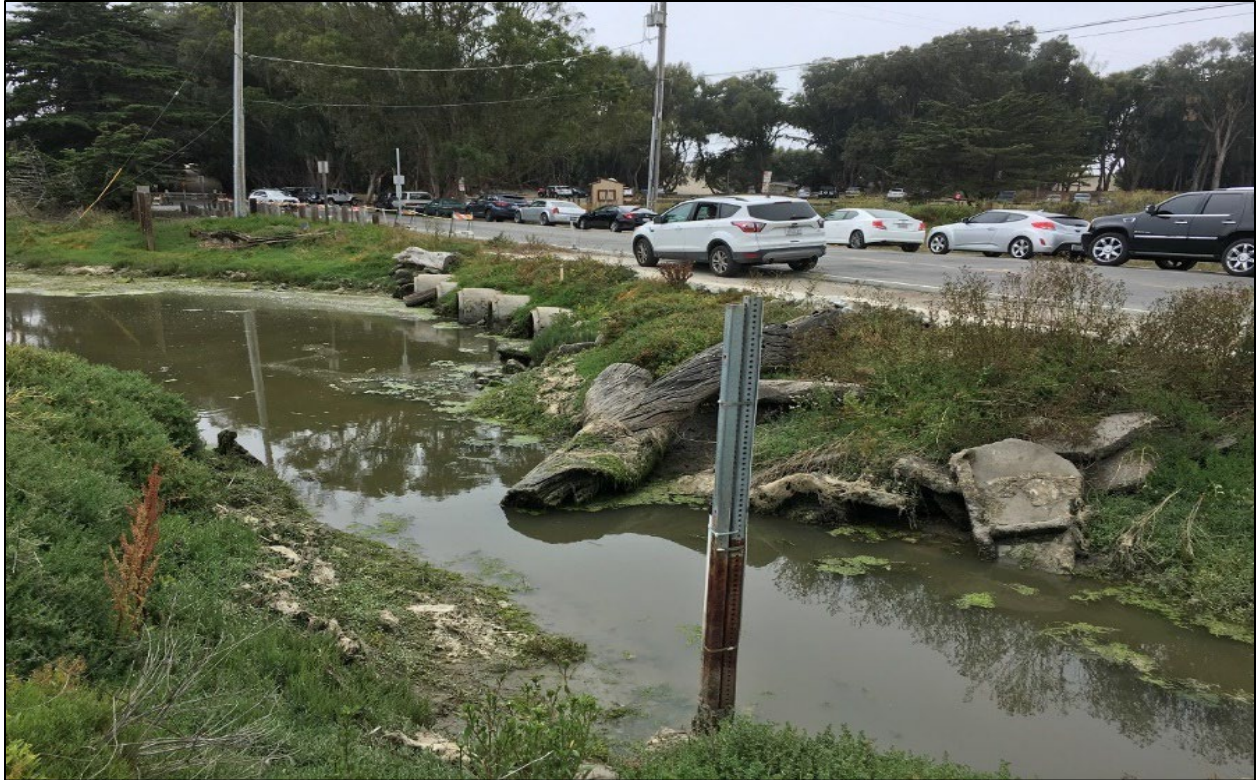
Figure 2-9. W. Beach Road Crossing and Culverts
