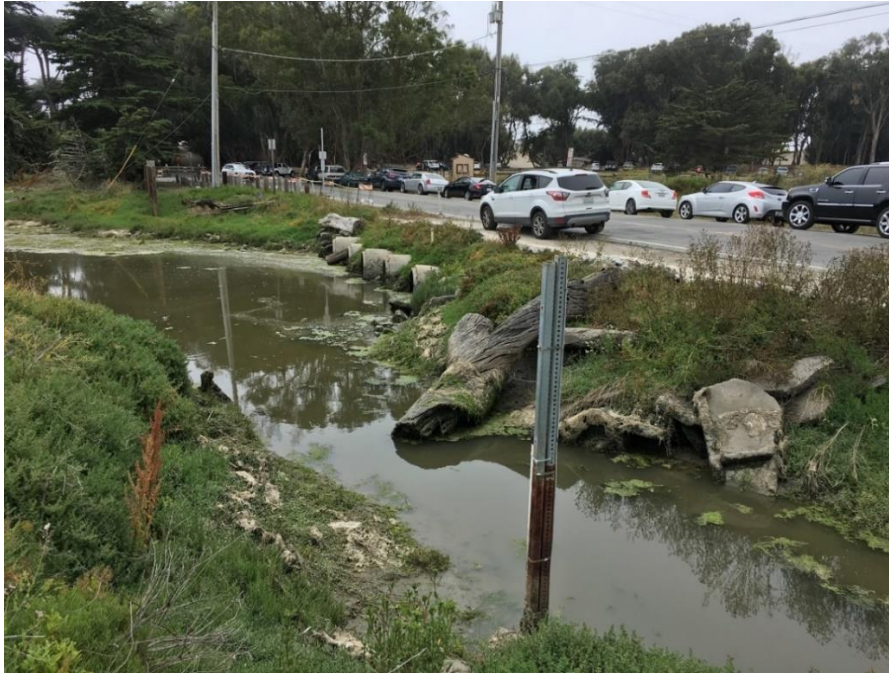
Figure 16: Beach Road crossing at Watsonville Slough – view of downstream side looking west.
