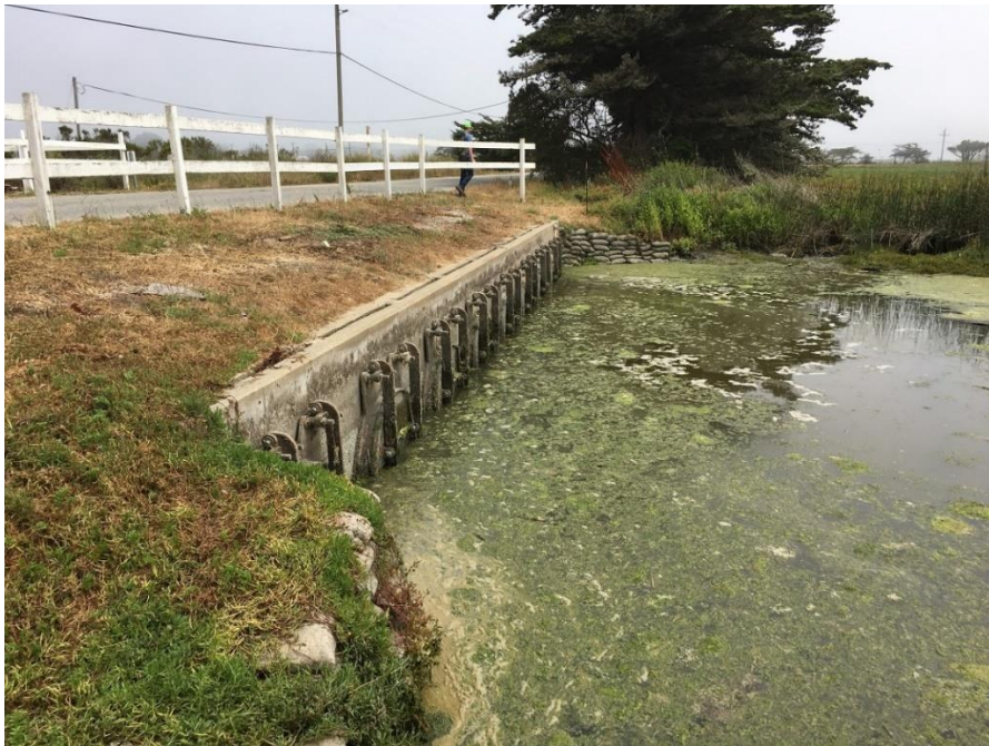
Figure 17: Shell Road crossing at Watsonville Slough – view of downstream side with 8 culverts with flap gates and vent array above the culverts.
