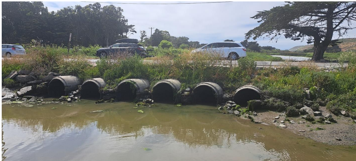
Figure 3 Photo looking upstream (N) at existing six (6) 48-inch diameter precast concrete culverts under West Beach Road
