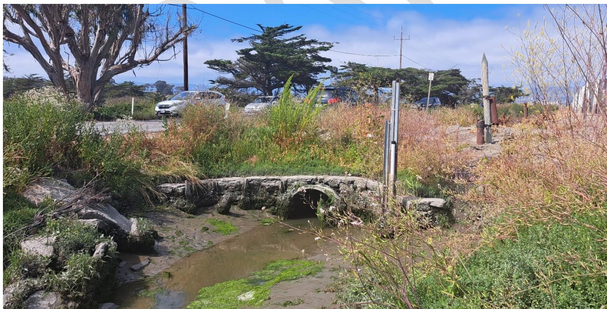
Figure 4 Photo taken from Slough channel, looking NE at the agricultural ditch outlet with existing 42" culvert and headwall.
