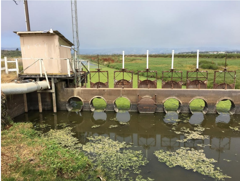
Figure 18: Shell Road crossing at Watsonville Slough – looking upstream from the road. View of pump station and old flow control weir.
