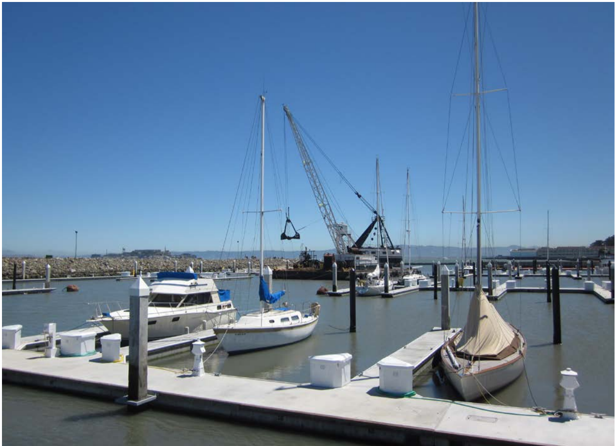
San Francisco Marina West Basin Maintenance Dredging 2013
