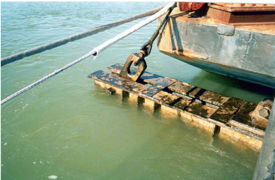
Figure 4. The knockdown bar suspended from the barge at the water surface.
