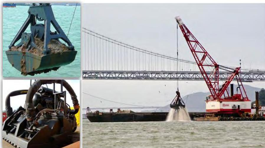
**Figure 2.** Top left: mechanical clam dredge (Photo: EIK Engineering), Bottom left: hydraulic dredge (Photo: Alibaba), Right: Dredging operation in SF Bay (Photo: Michael Slater).
