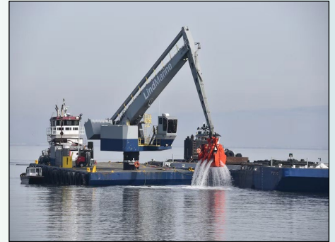
USACE Clamshell Dredge in San Francisco Bay
