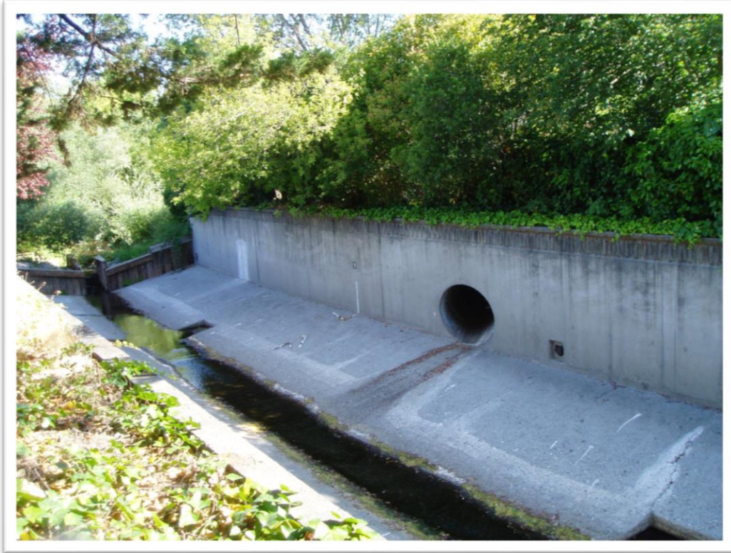
Photo 4.1-A. View of the storm drain outfall downstream of the Denil fish ladder
