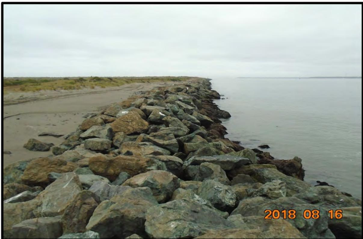
Figure 6. Photo of entire jetty cross-section in need of repair (Type 3).
