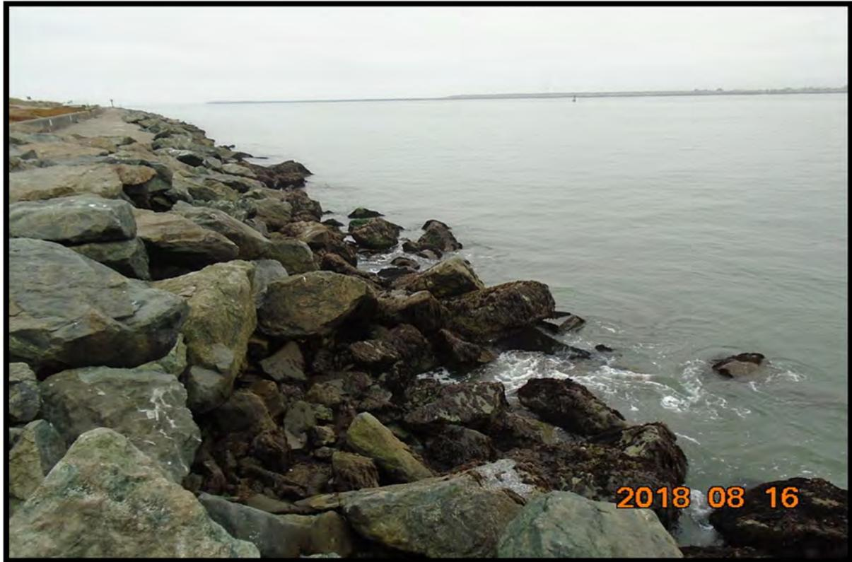
Figure 5. Photo of jetty slope in need of repair (Type 2).
