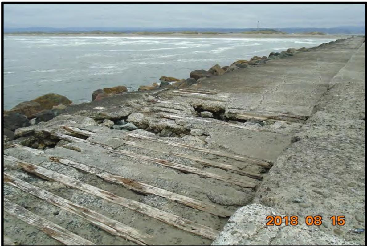
Figure 4. Photo of concrete cap in need of repair (Type 1).
