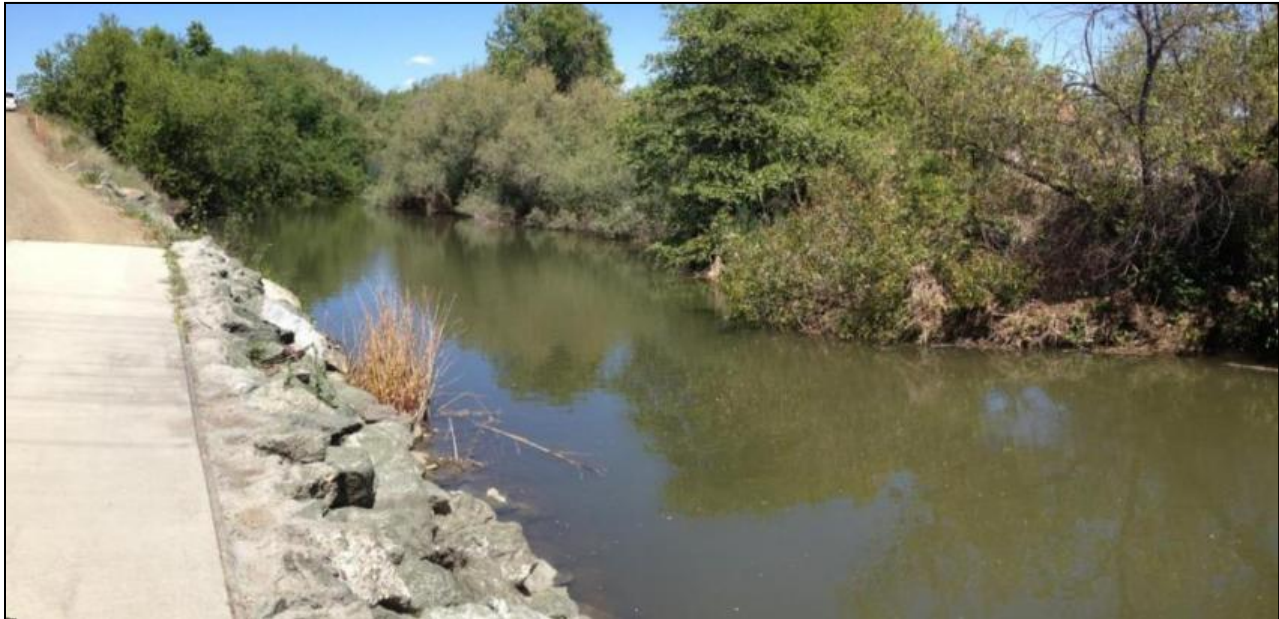
Figure 9. Site 1 – Gravel Augmentation Site from Stations 1018+00 to 1004+00 (Looking downstream at backwater pool. Proposed conversion to a low gradient riffle)
