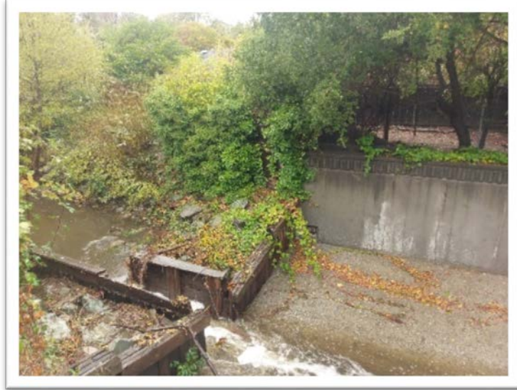
Photo 1. Denil Fish Ladder from the Right Bank (taken November 2017)
