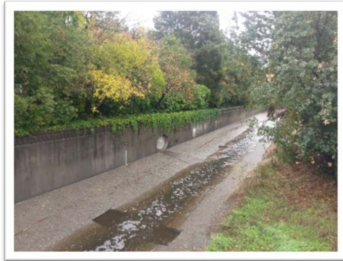
Photo 3. Concrete Channel Downstream of the Fish Ladder taken from the Right Bank
