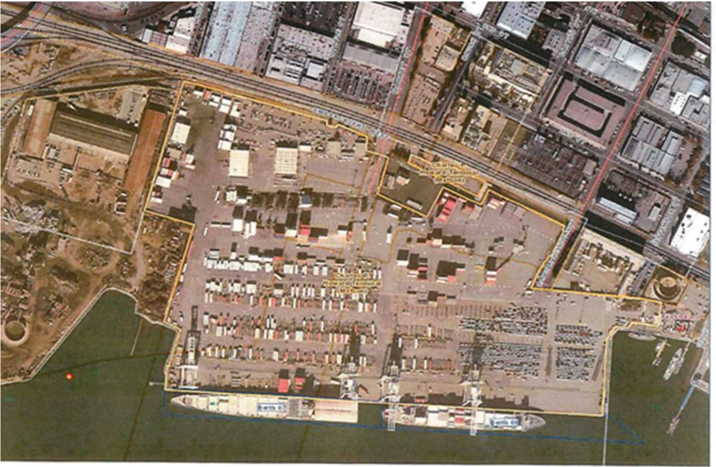
Figure 8-5: View of Howard Terminal Facility/Utility Footprint
