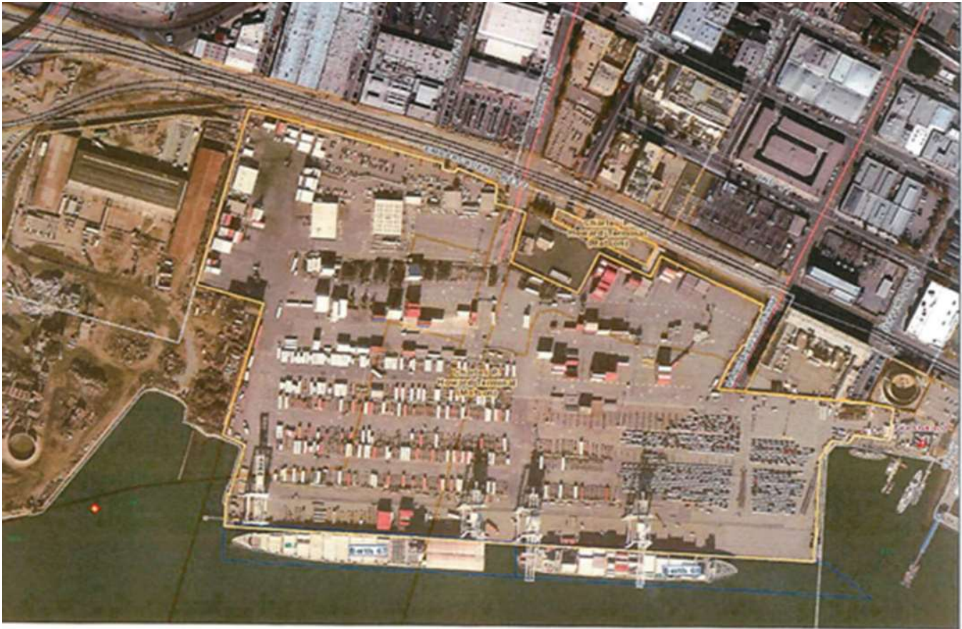
Figure 16-1: View of Howard Terminal Facility/Utility Footprint
