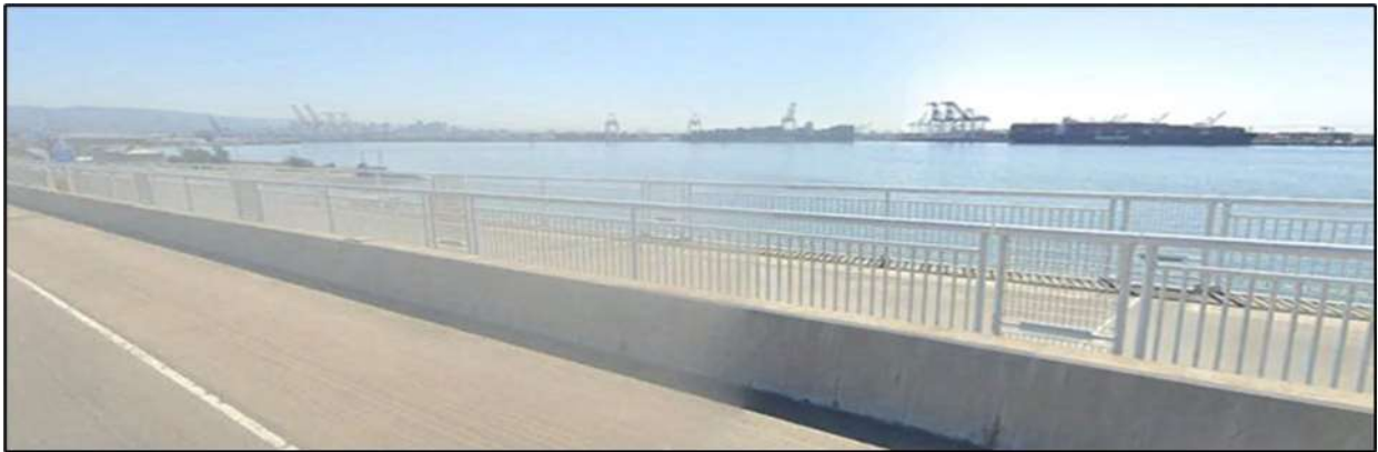
Figure 2-3: View of the Outer Harbor Turning Basin from the Bay Bridge Looking East
