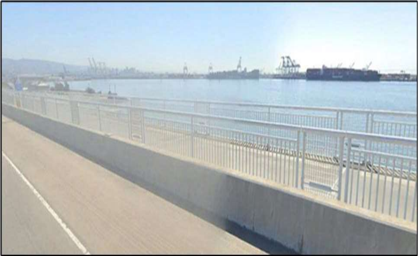
Figure 8-3: View of the Outer Harbor Turning Basin from the Bay Bridge Looking East
