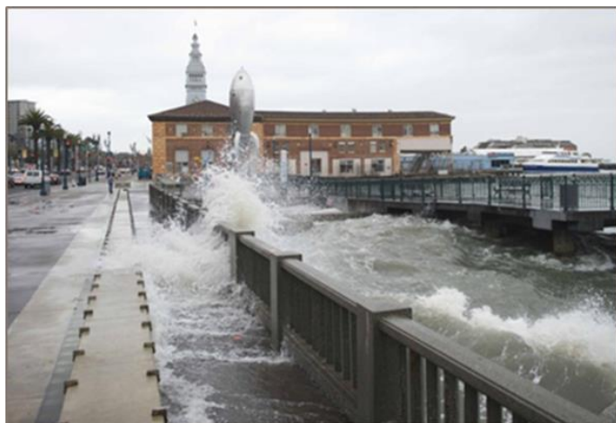
Figure 2: Overtopping of the seawall along the Embarcadero roadway and pedestrian promenade south of the Ferry Building
