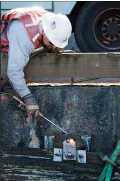
[Left] A Port of San Francisco employee uses a blow torch to cut through metal supports holding a deteriorated piling to Pier 23. [Above] The new James R. Herman Cruise Terminal will house the America's Cup headquarters during the race—Sept. 7-21, 2013. [Right] Richard Curry uses the Dillard's pedestal-mounted grapple crane to lift a rotted piling from the bay onto the Dillard's deck.
