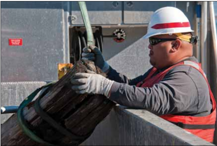
Ray Santos, a Dillard crew member, removes lines and secures a rotted piling on the deck of the Dillard. The collected pilings, along with other debris, are taken to Sausalito, Calif., where they are stored and then disposed of.
