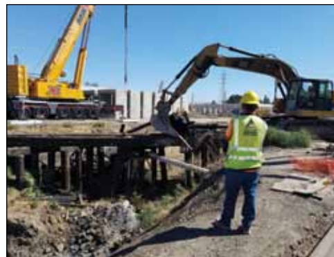
Crews demolish the old trestle bridge [right], while installing a series of box culverts [above] at Berryessa Creek in Milpitas Oct. 2.
