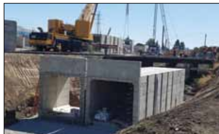
Crews demolish the old trestle bridge [right], while installing a series of box culverts [above] at Berryessa Creek in Milpitas Oct. 2.
