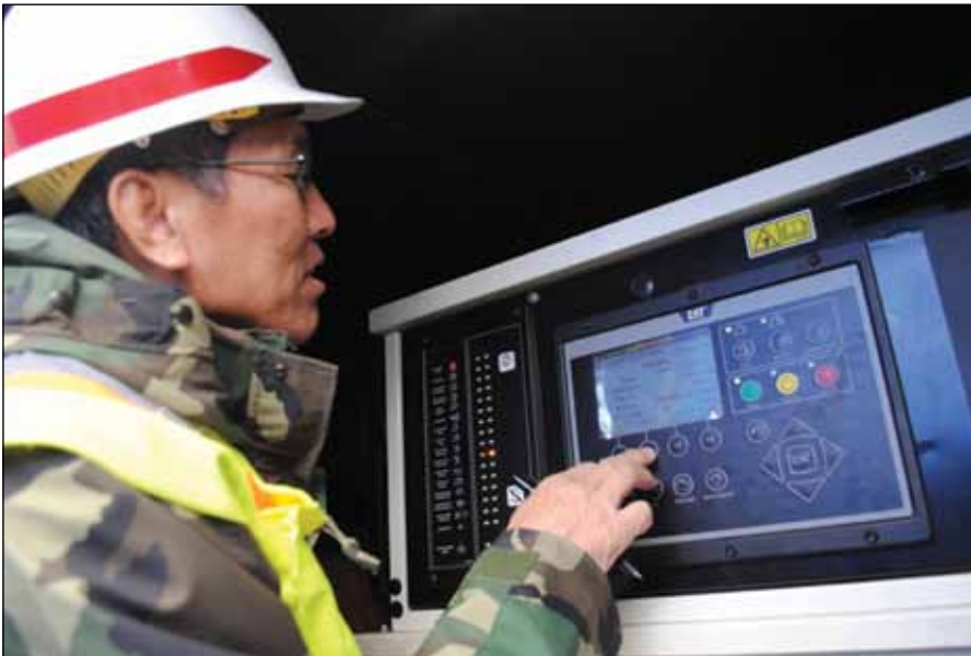
Elton Choy of the USACE Honolulu District inspects an emergency generator in Queens, N.Y.
