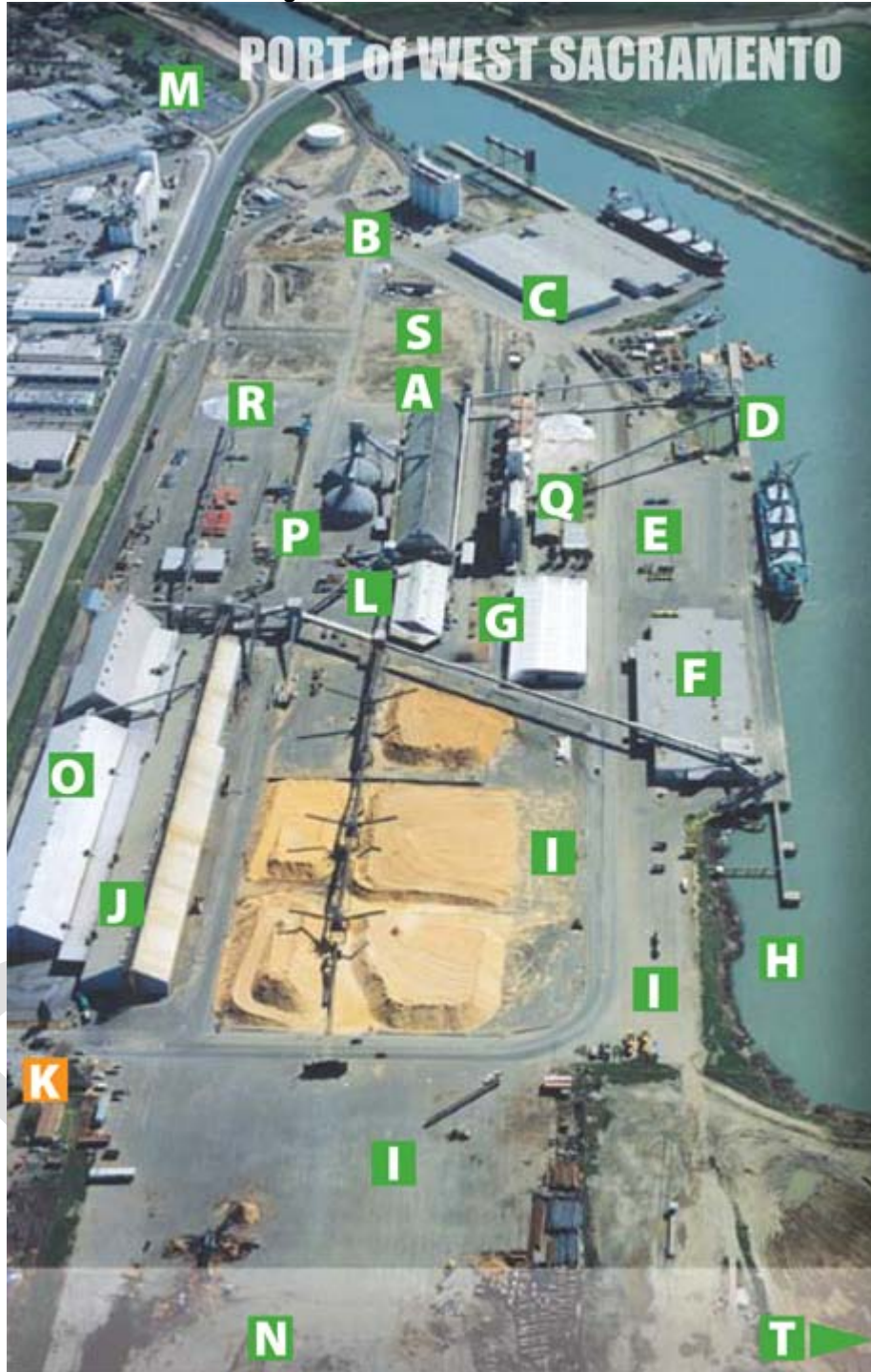
Figure 2: Aerial of Port Facilities 4
