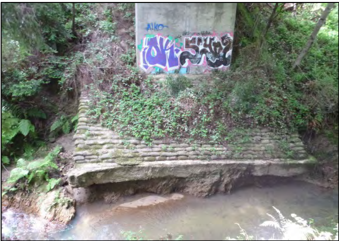
Photo 4. Scouring evident at the base of Cloverdale Road bridge. Erosion protection improvements are needed.
