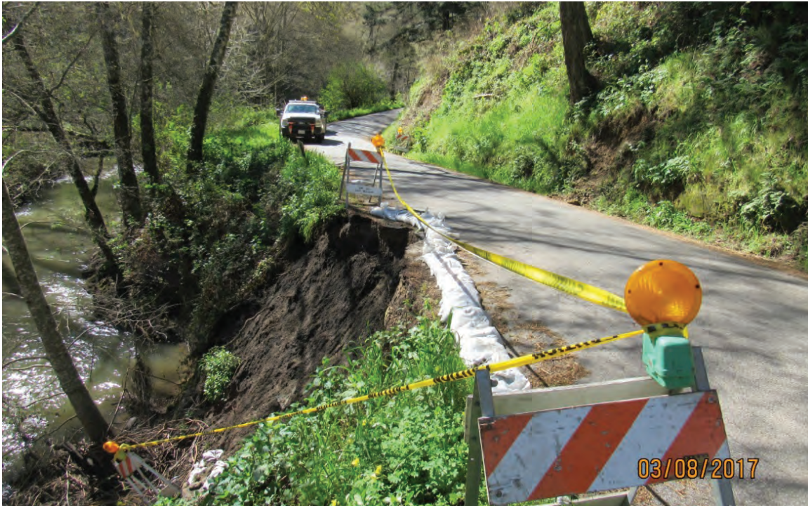
Photo 3. Example slope failure along Gazos Creek and Gazos Creek Road. This site was addressed in the County's 2017 emergency permit application. (March 2017)
