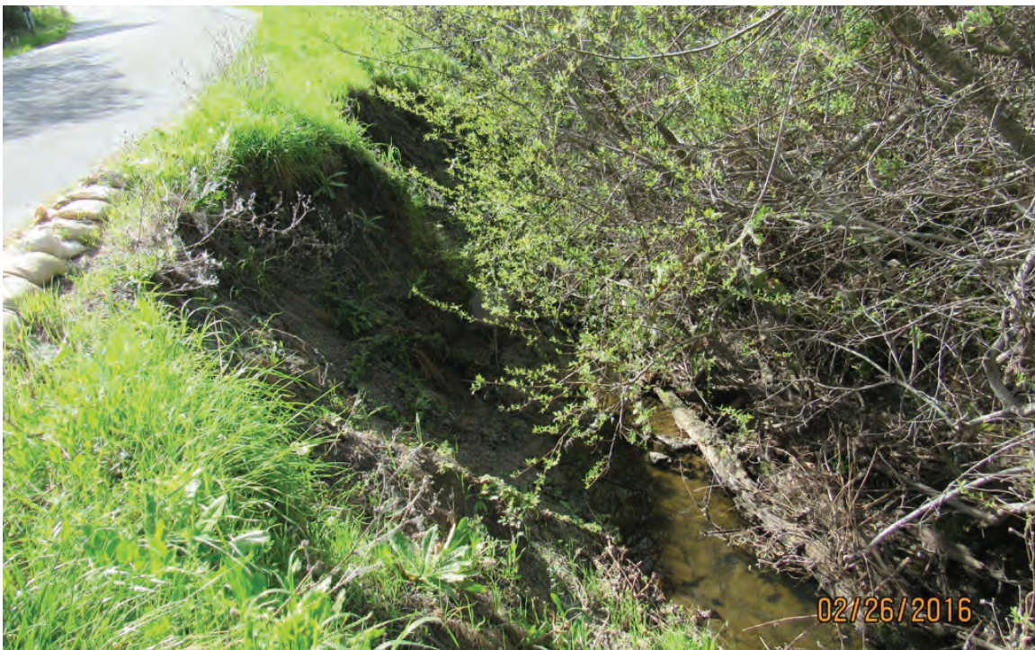
Photo 2. Bank failure along Lower Bear Gulch Road and adjacent to Clear Creek, an intermittent tributary to San Gregorio Creek. (February 2016)
