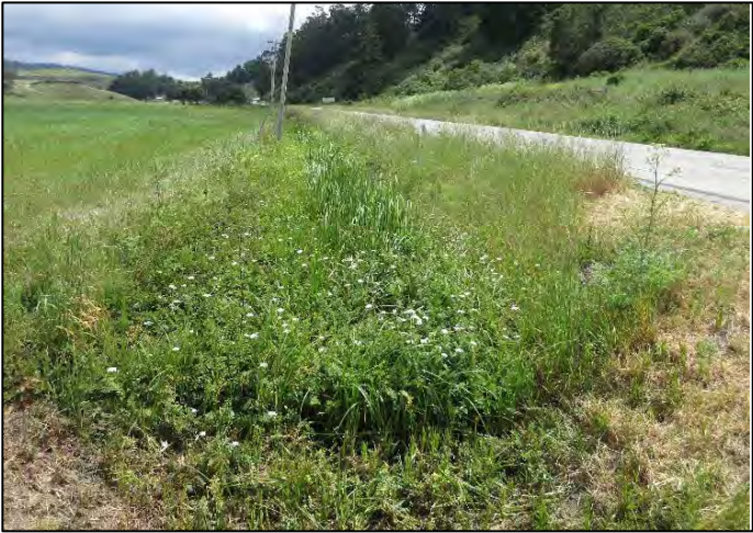
Photo 10. Unpaved ditch along Cloverdale Road in Pescadero. Potential need for sediment and vegetation removal in the future. (May 2015)
