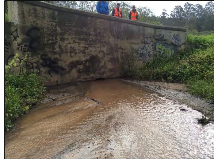
Photo 6. Upstream side of George Street bridge where substantial sediment accumulation has occurred and is blocking the culvert (April 2017)
