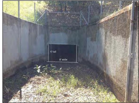
Photo 2. Pine Creek box culvert (downstream end). No flow present at time of survey. (April 2014)
