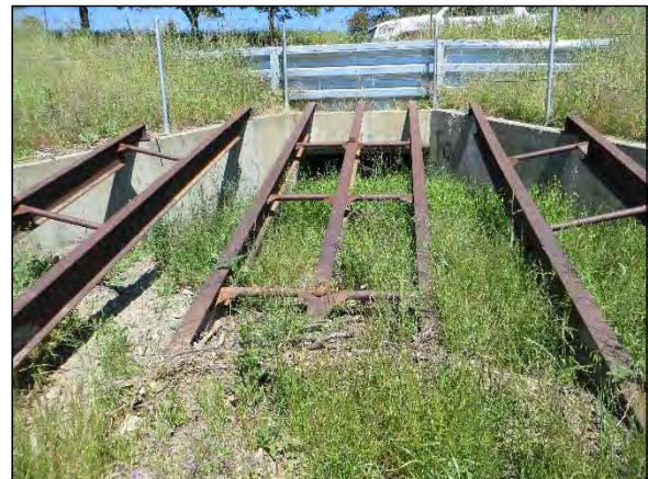
Photo 4. Metal trash rack covering entrance of upstream end of Pine Creek box culvert. (April 2014)
