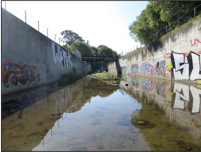
Photo 1. U-shaped concrete channel. View of San Pablo Creek looking upstream near Parr Boulevard in Richmond. (April 2014)
