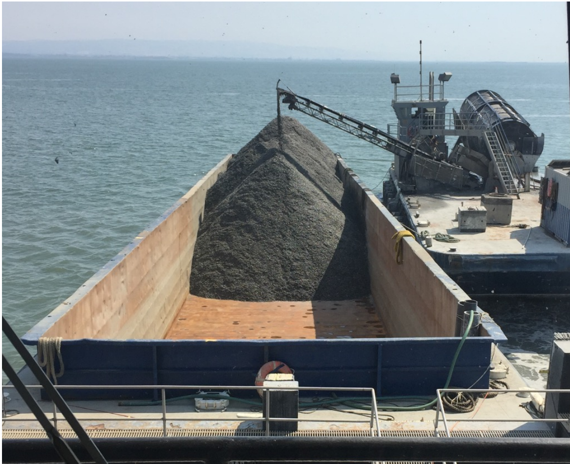
Figure 1-4: New Shell Dredge Engaged in Dredging
