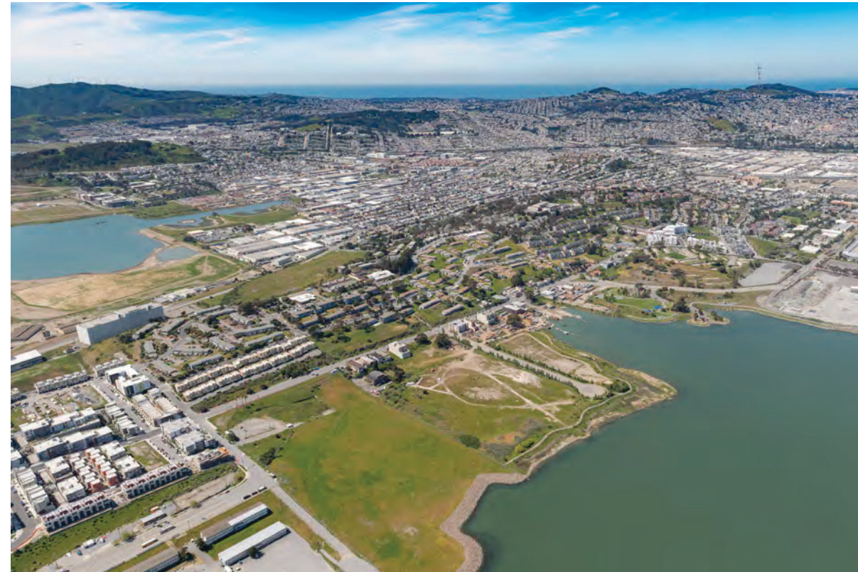
View facing West
