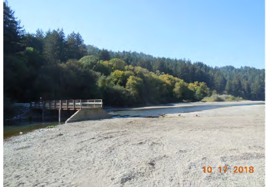
Photo 3. Crossing removed and closed for winter season, 2018.
